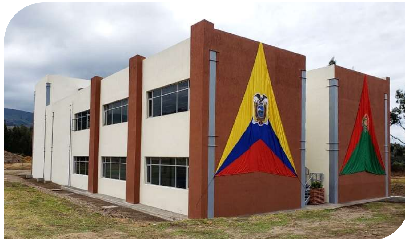
● ESPE ELECTRICAL AND ELECTRONIC LABORATORY BUILDINGS – LATACUNGA. University campus.
