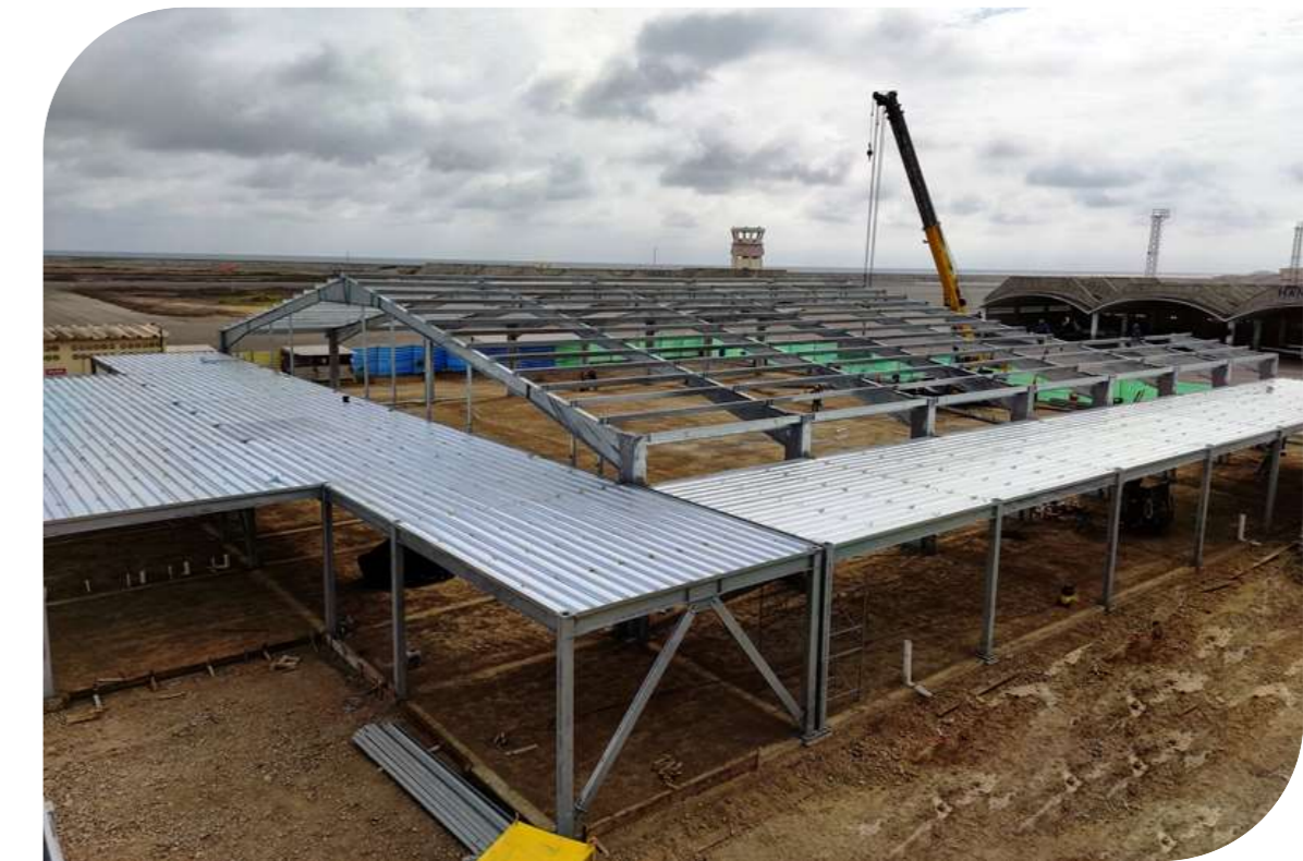
● FAE SALINAS Construction of the Aircraft Shelter
