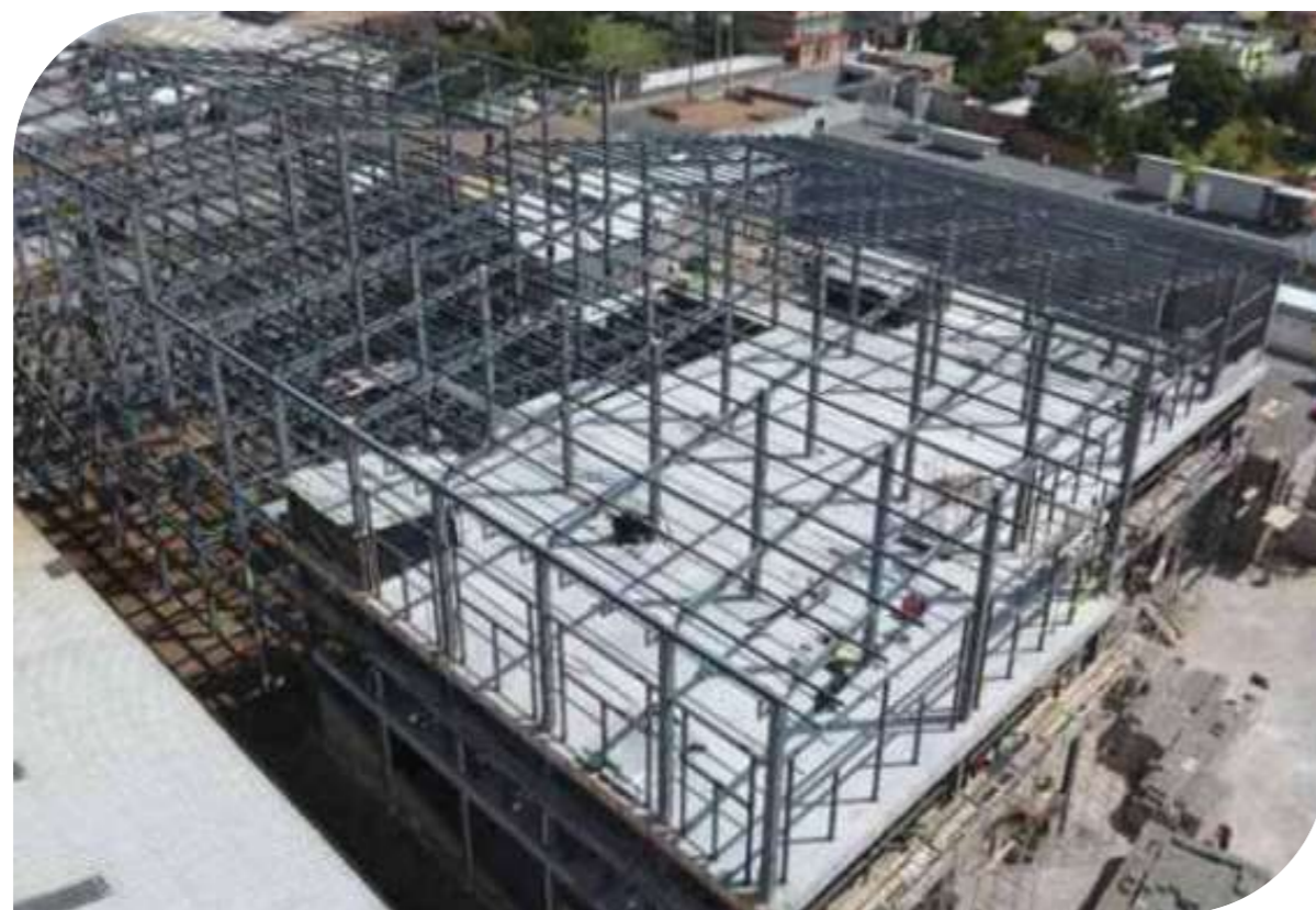
● NILOTEX Construction of the Production Plant.
