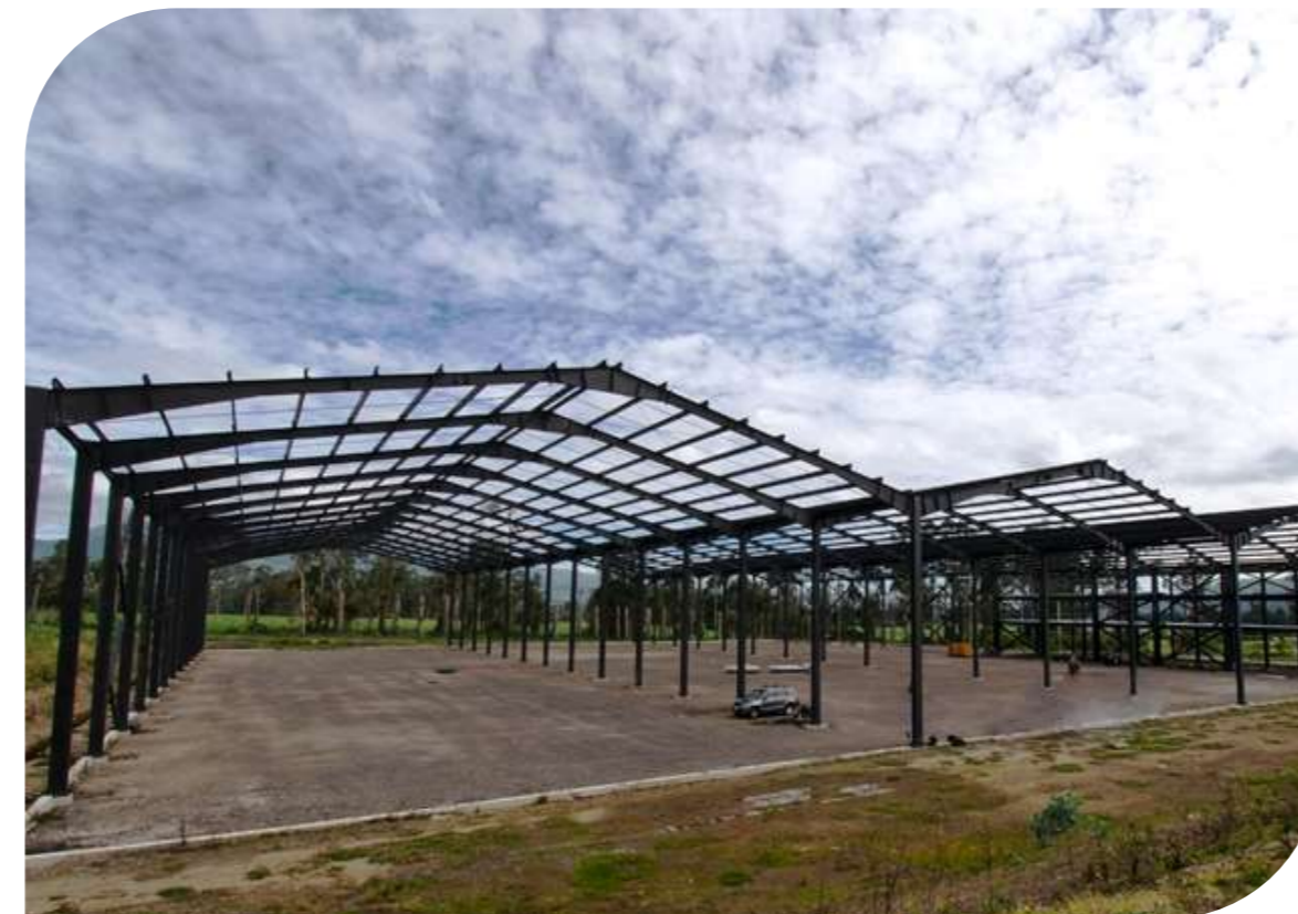
● UMCO ECUADOR Construction of the Industrial Plant and Logistics Center.
