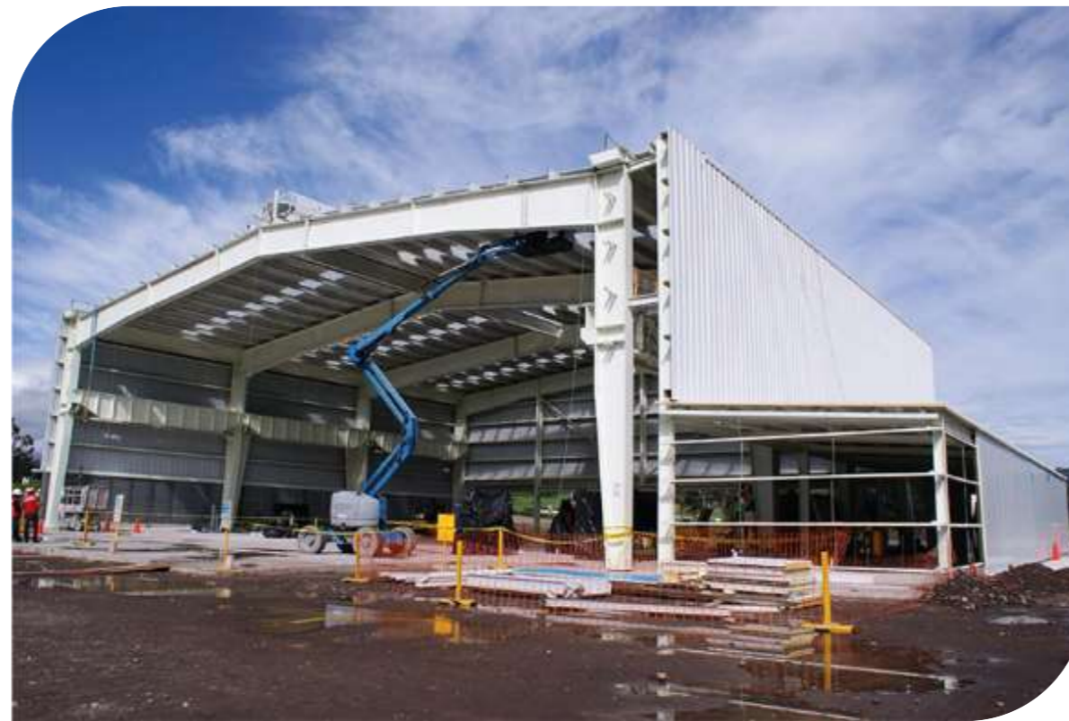
● TENARIS Construction of the Industrial Plant
