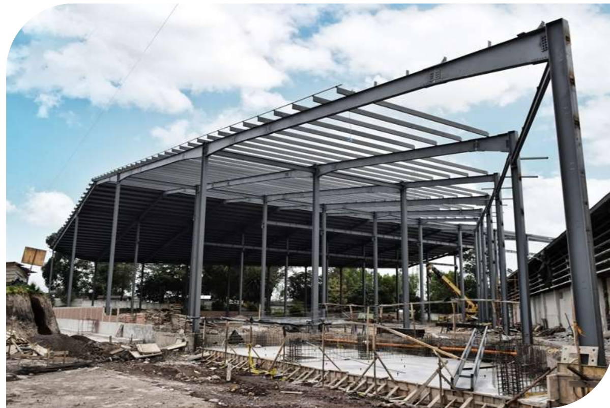
● CHAIDE & CHAIDE Construction of the Industrial Plant.
