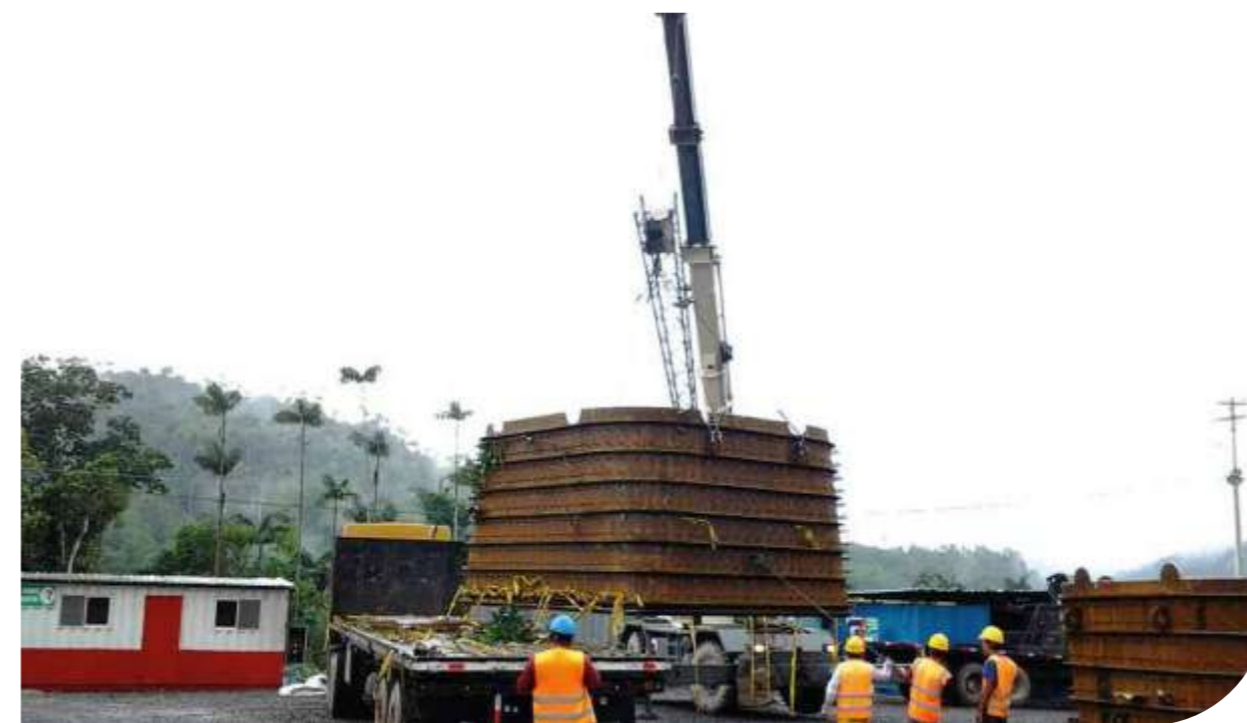
● HIDROELECTRIC PLANT MANDURIACU Transition and Drain Shielding
