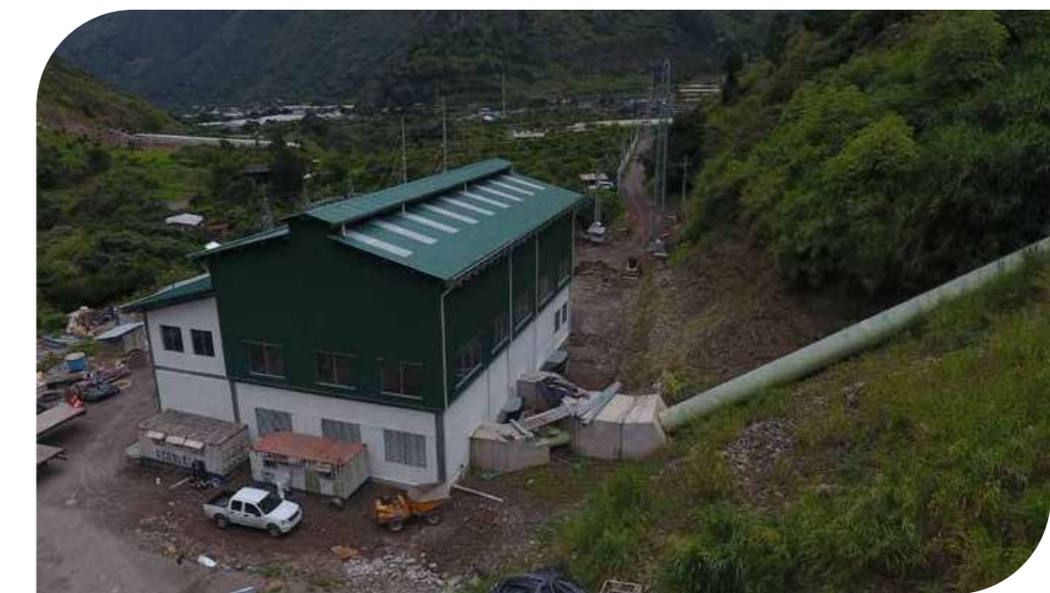
● HIDROELECTRIC PLANT HIDROSIERRA Machines House and Pipes
