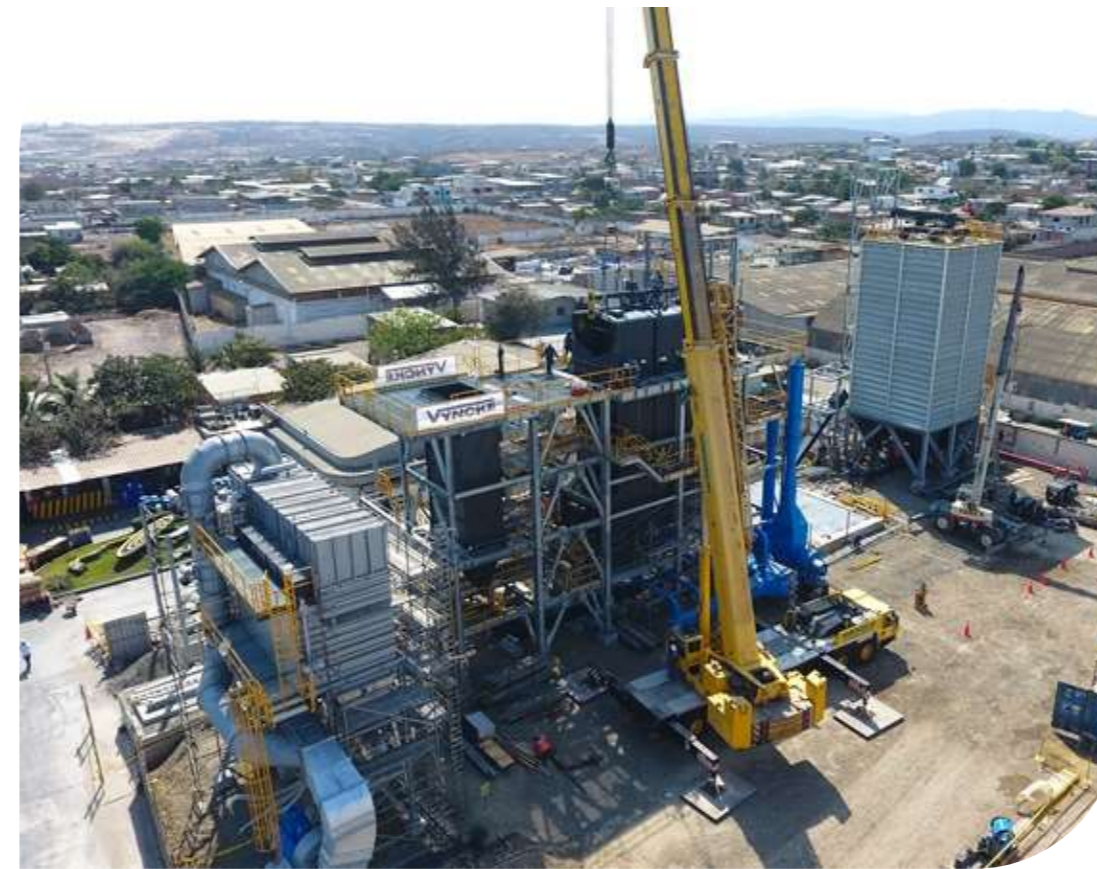
● LA FABRIL Biomass Plant Construction
