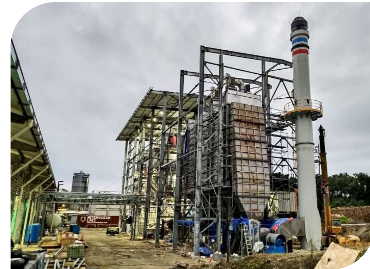
● BOTROSA Biomass Plant Construction
