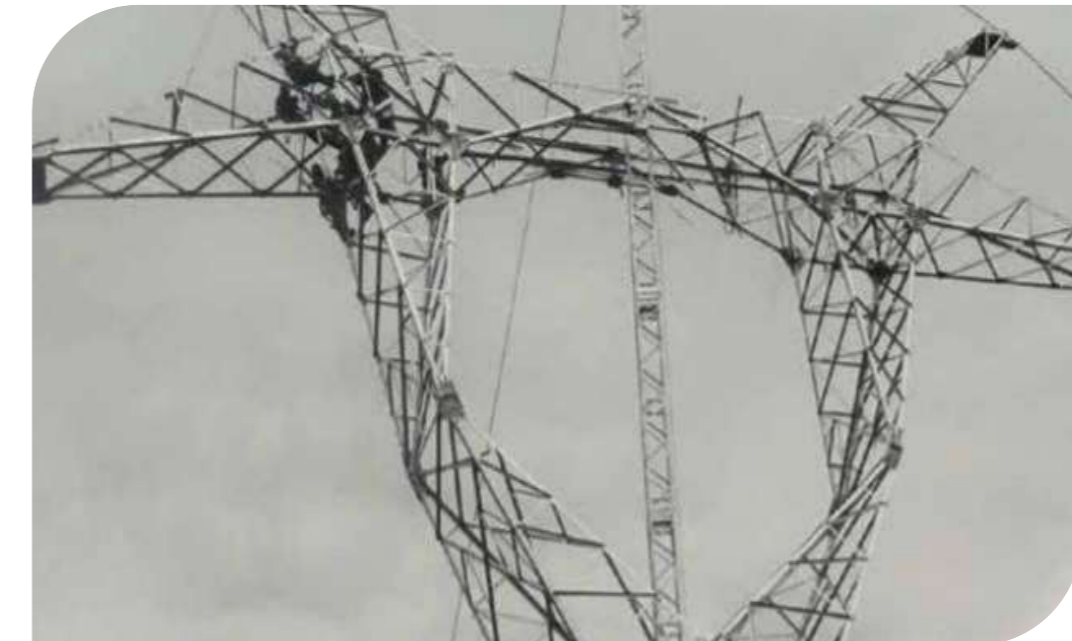
● San Rafael Transmission Line - El Inga 500kV Substation
