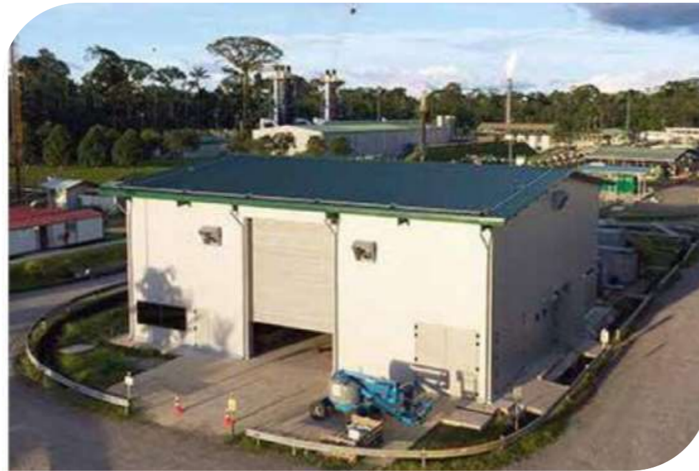
● Block 12 – PAM Maintenance Workshop
