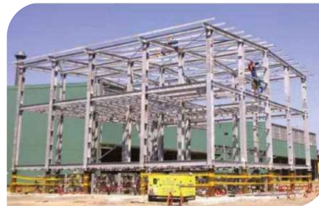
● SHINA OGE Electrical Building
