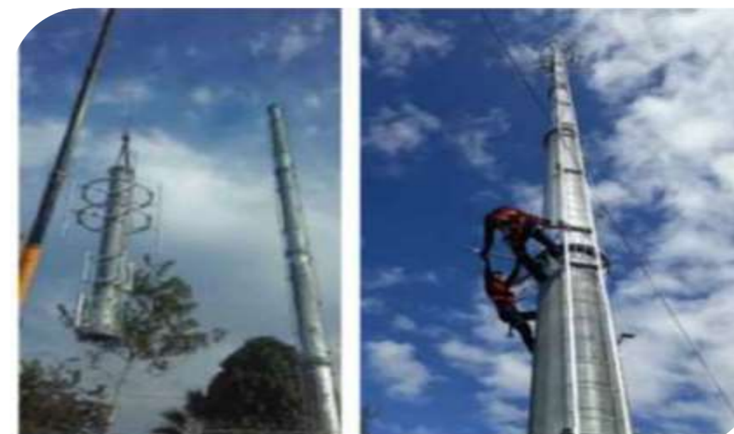
● Supply of Structures for Towers 2017 - 2018
