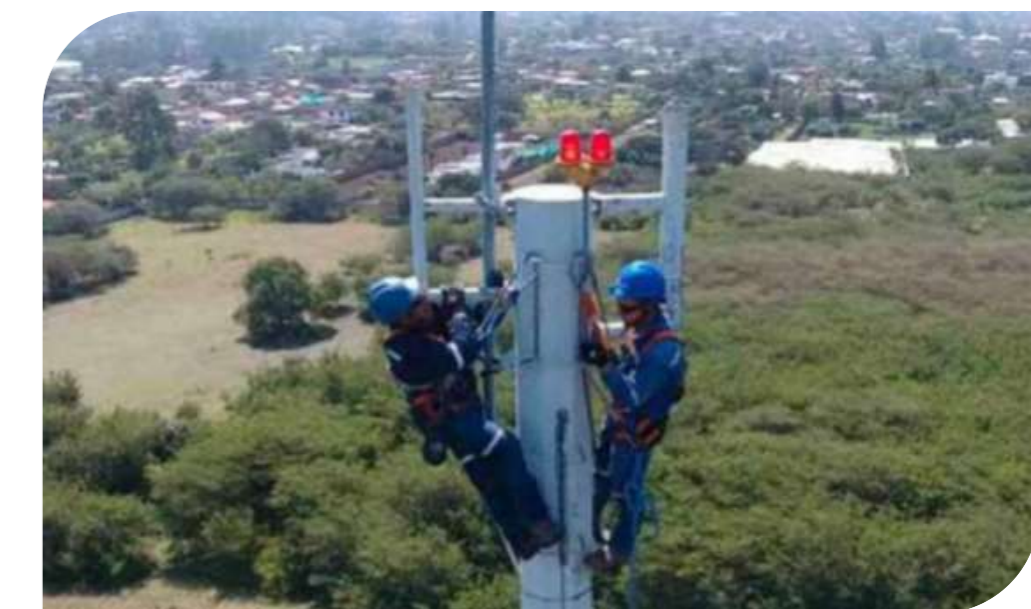
● Maintenance of Towers and Monopoles.
