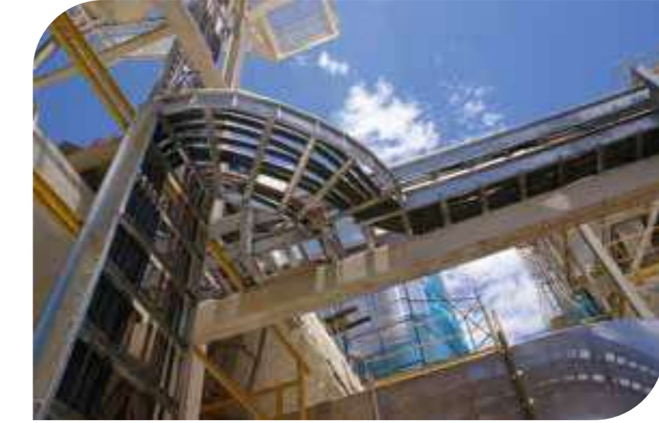
• Novopan Industrial Plant Repowering 2.500 m of pregalvanized trays.
