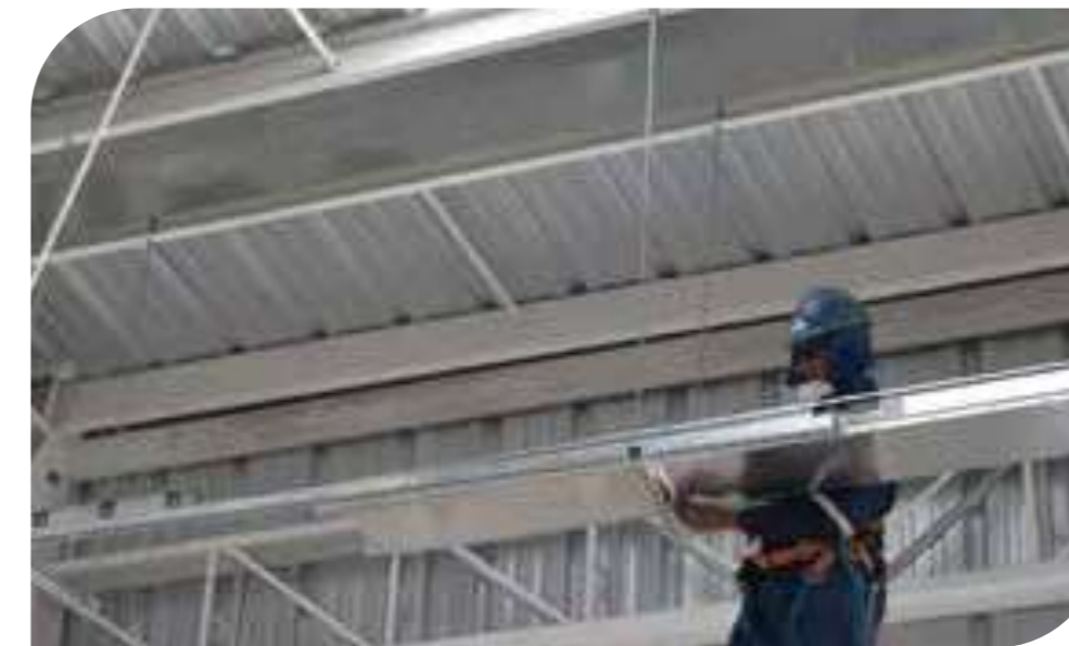
• FV Área Andina Plant 600 m of aluminum trays.
