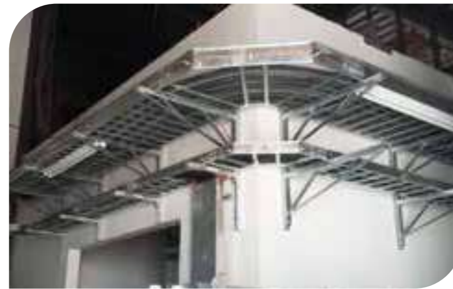
• Cuenca Tram Substation. 100m of galvanized trays.
